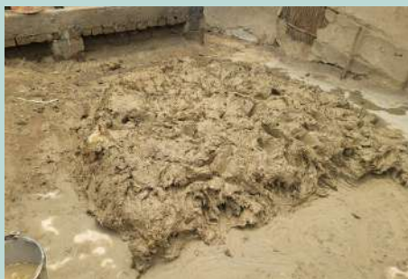
Mud mixed with husk and cow dung was applied to bamboo walls in Jeetpursimara to enhance insulation.
