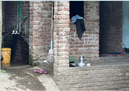
Sprinkled water on floors and walls.
