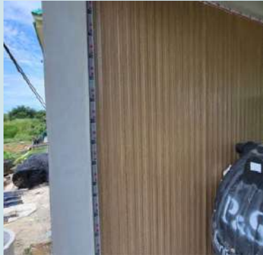
Insulated metal sheet "sandwiches" as walls.
