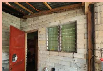
Windows with adjustable louvers in this house in the Philippines allow air to flow in.
